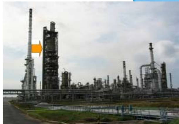
Existing Thermoform Catalytic Cracking Unit (TCU) at the Bataan Refiner
